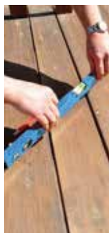
Turn the level 180° side to side
